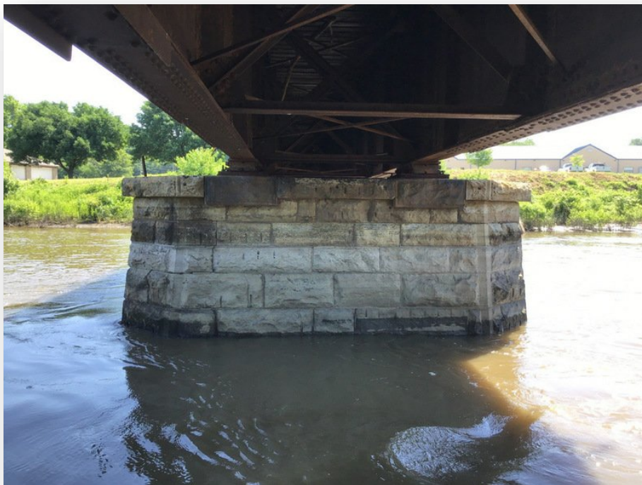
Figure 9 - Pier 25, Downstream Bullnose
