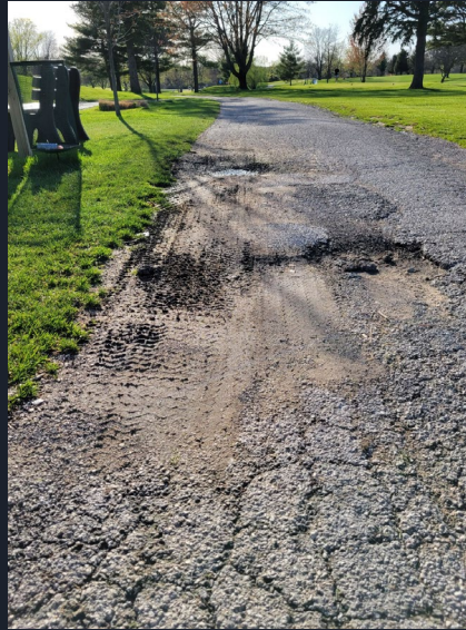
Areas of the paths have large potholes, which makes for a poor ride experience.
