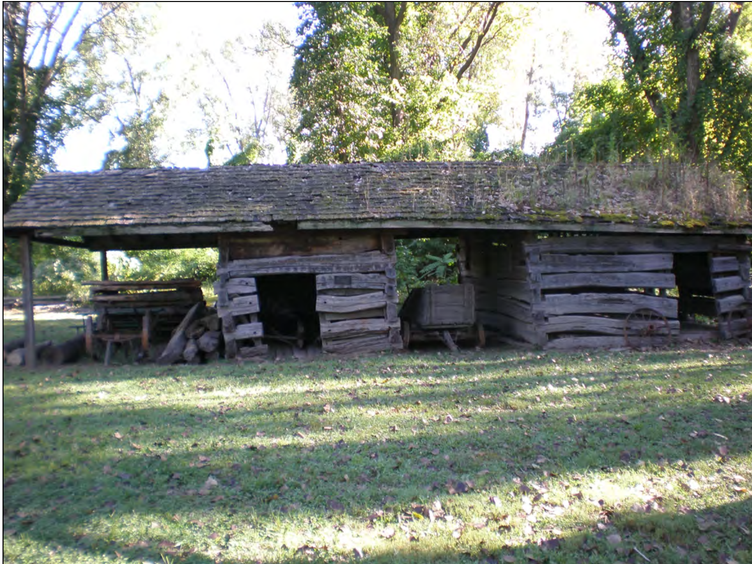
Figure 10. Corn Crib. This image shows the 2 pens as they lean to the north. The roof has exceeded its useful life, and two pens contain material that should be disposed of appropriately.
