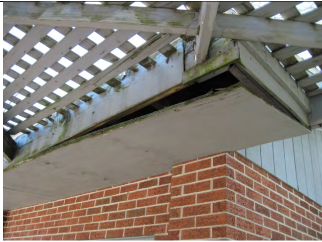
Soffet Water Damage
