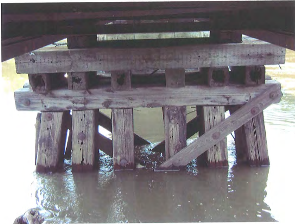
Photo No. 75 Looking east at timber lagging under span 5.
