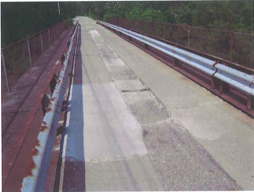
Photo No. 15 Looking west at full depth concrete repair.
