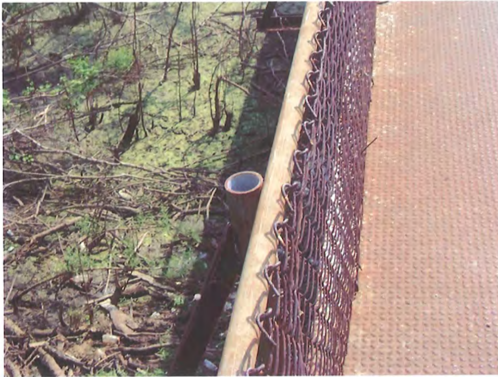
Photo No. 19 Looking at a loose pedestrian rail connection.
