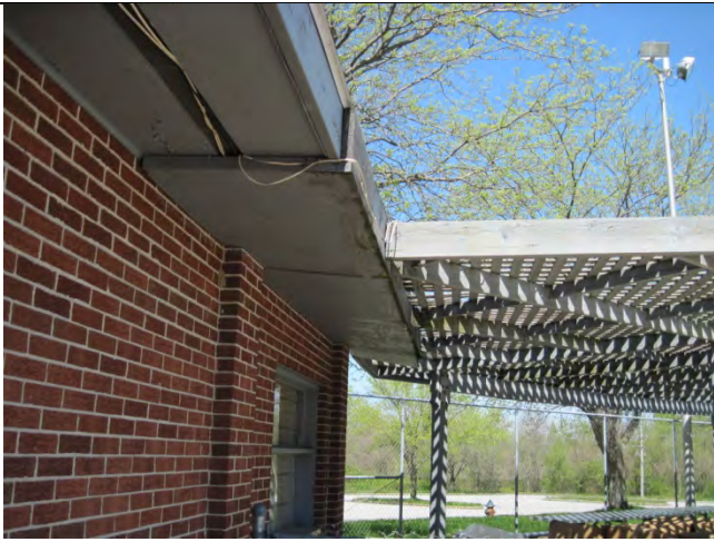
Soffet Water Damage
