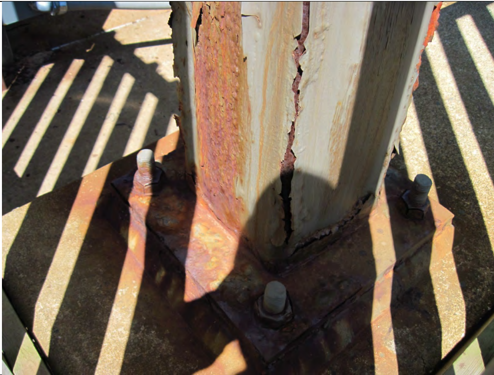
Support Deterioration
