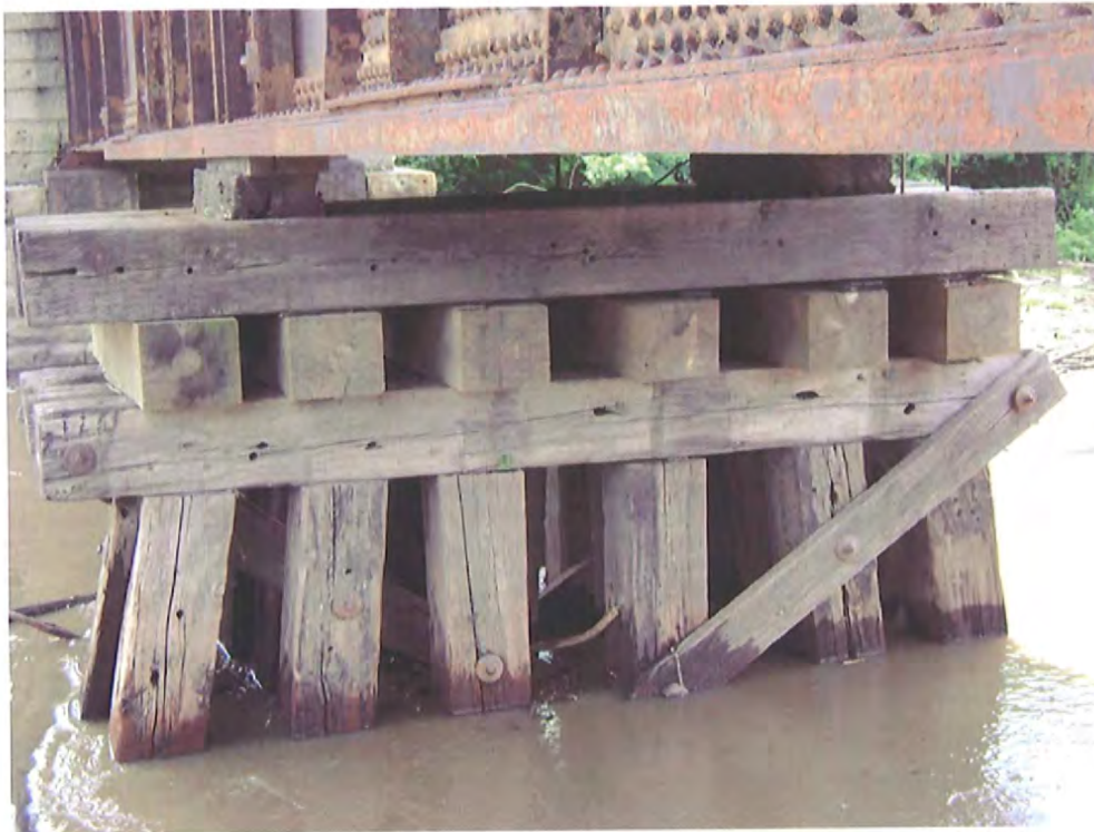
Photo No. 76 Looking east at timber lagging under span 6.
