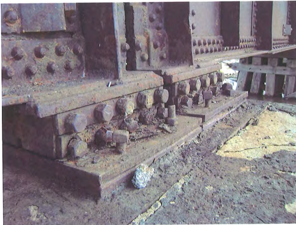
Photo No. 64 Looking east at south girder bearings, pier 5.
