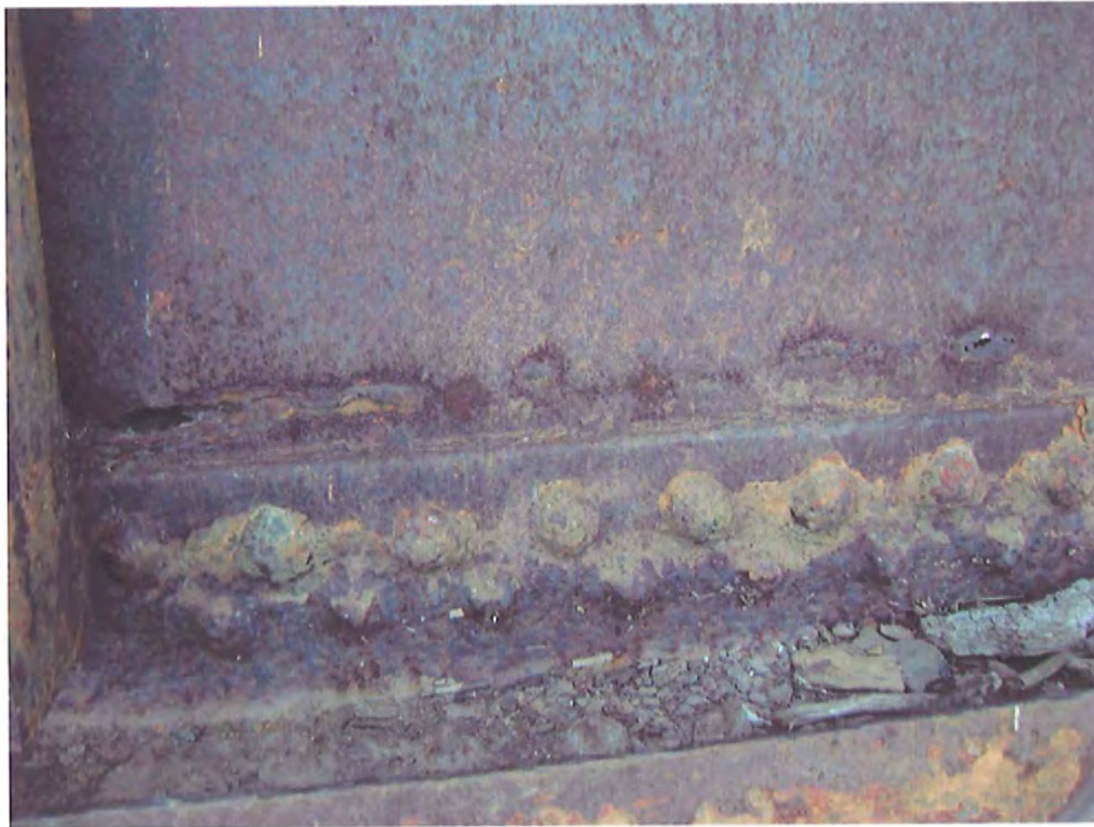
Photo No. 53 Looking at web deterioration of south girder, span 4.
