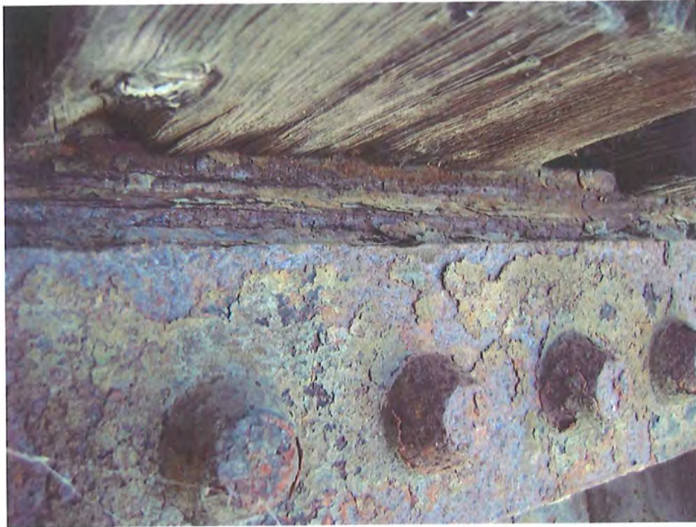
Photo No. 41 Looking at pack rusting at the top flange splice of south girder, span 3.
