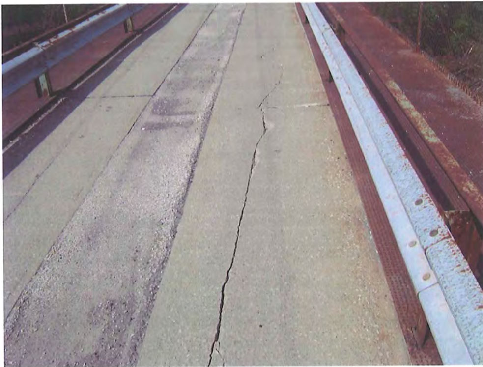
Photo No. 16 Looking west at typical longitudinal cracking.
