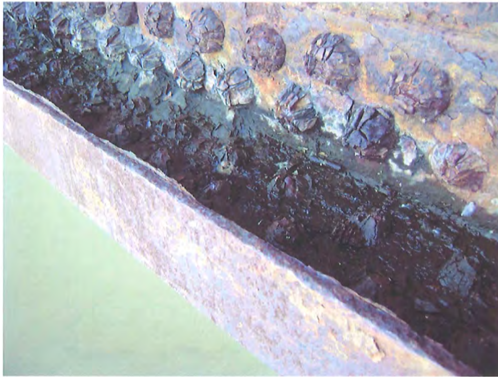
Photo No. 49 Looking at deteriorated rivets at bottom flange of north girder, span 4.
