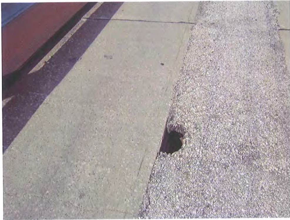
Photo No. 14 Hole through deck the near the middle of the structure.
