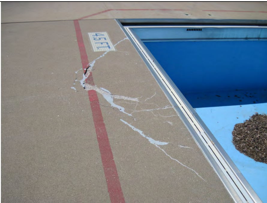
Deck Cracking
