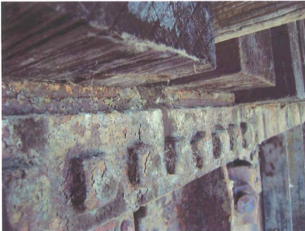
Photo No. 46 Looking at top flange splice of north girder, span 4.
