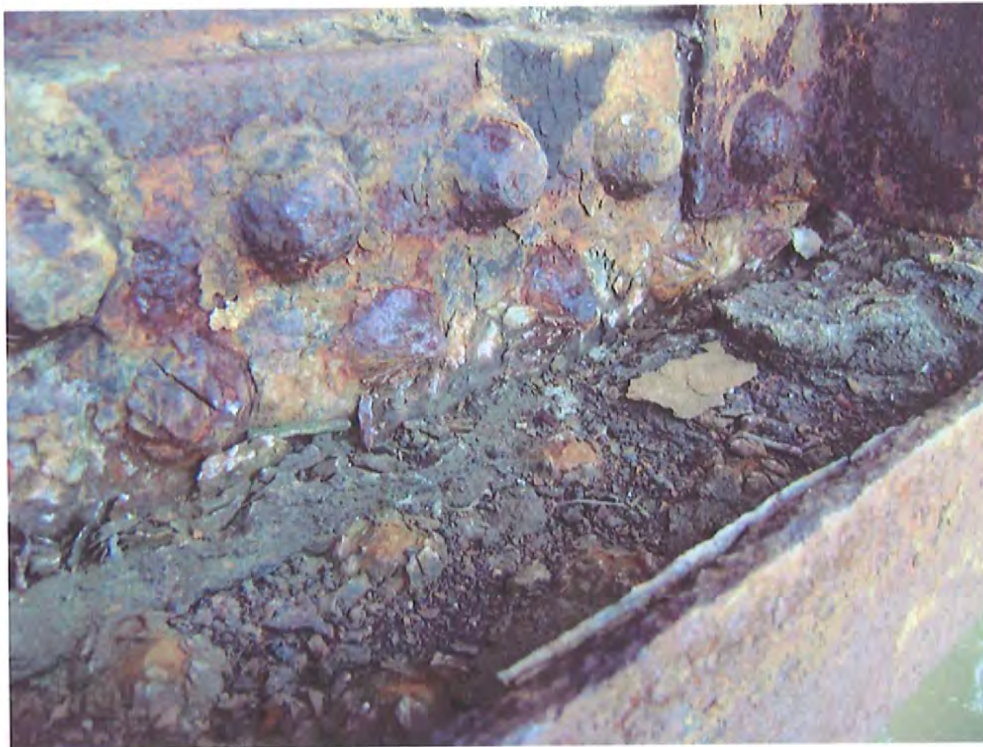
Photo No. 42 Looking at deterioration of rivets, north girder, span 3.
