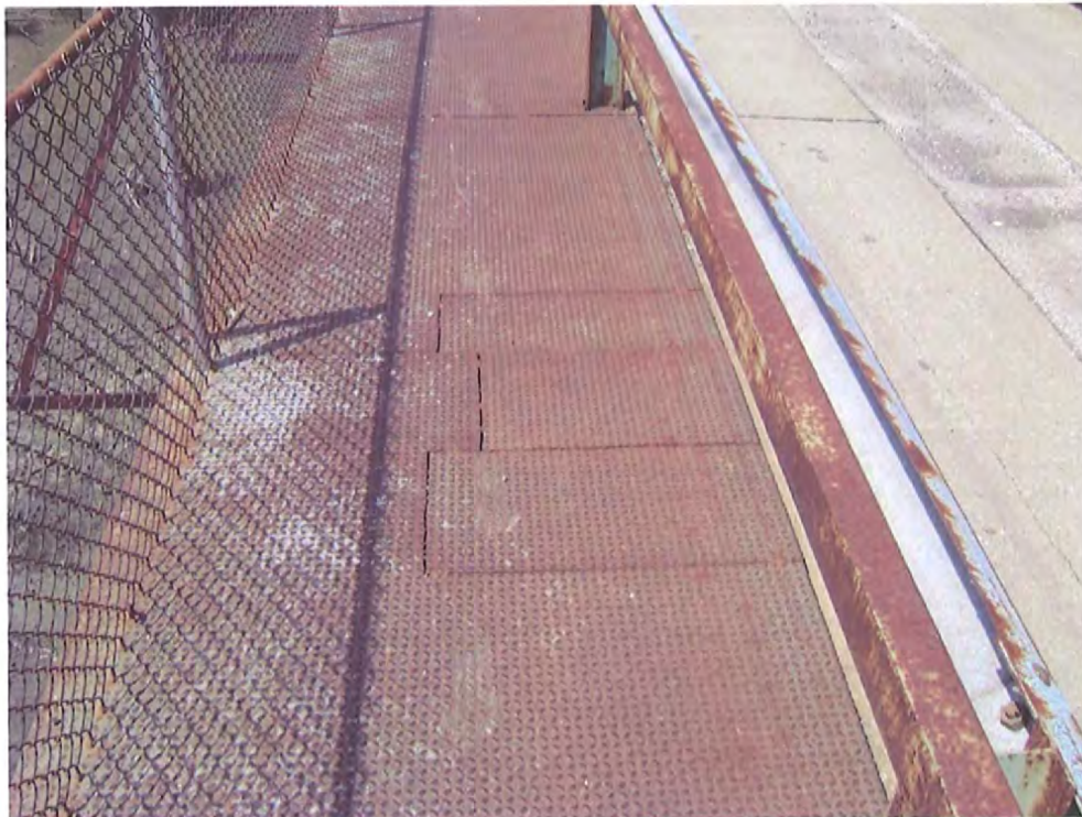
Photo No. 22 Looking at maintenance access areas in checkered plating
