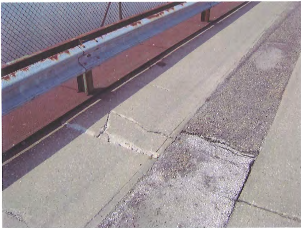
Photo No. 20 Looking southwest at typical transverse cracking in deck.
