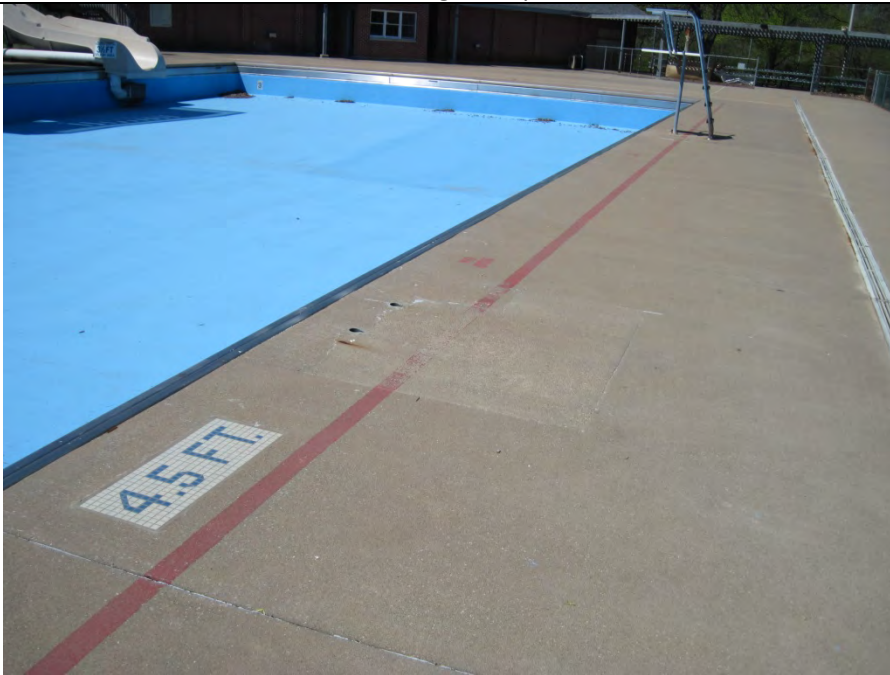
Deck cut to repair filtered water pipe failure
