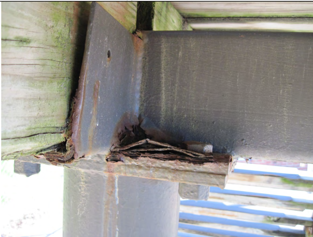
Step Support Deterioratoin
