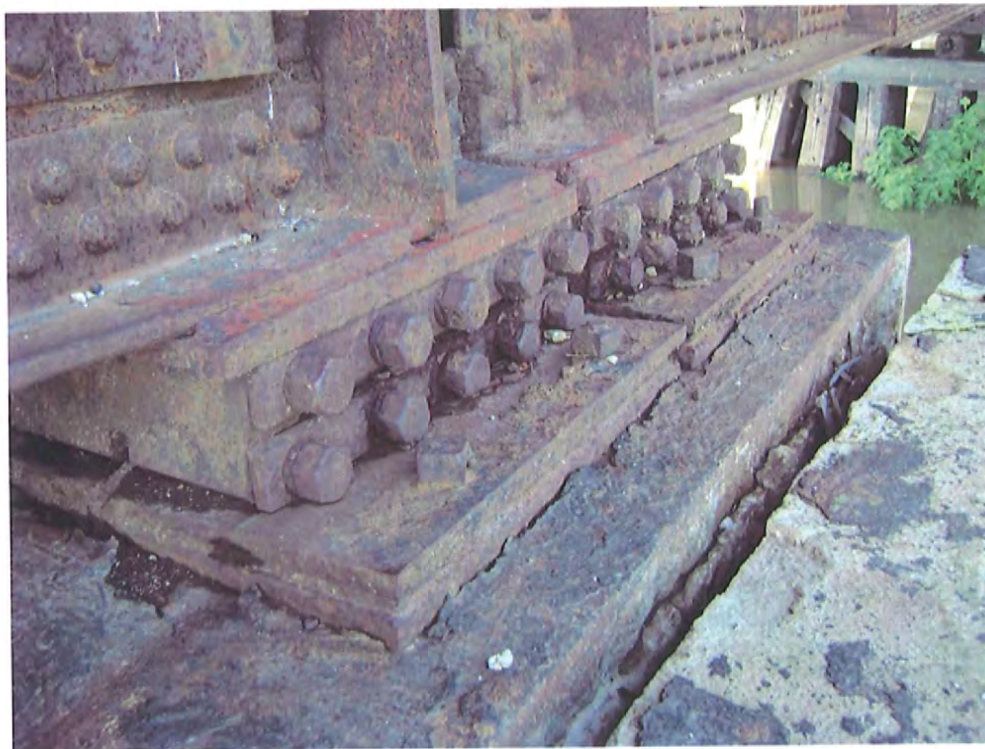
Photo No. 28 Looking southwest at north girder bearings, pier 1.
